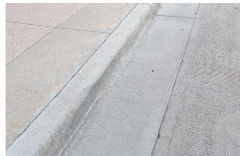
Type A Curb and Gutter
